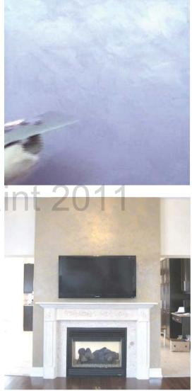
The overall area of application should be divided into manageable areas respecting expansion joints, divide up into zones. This is particularly recommended for the less experienced user. Protect adjacent areas and floors, to remove dry product use warm water or mineral spirit, do not rub with abrasives.
